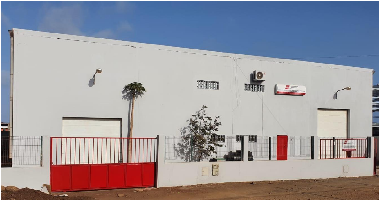
AGS Cape Verde's new facilities following a four-month renovation.
